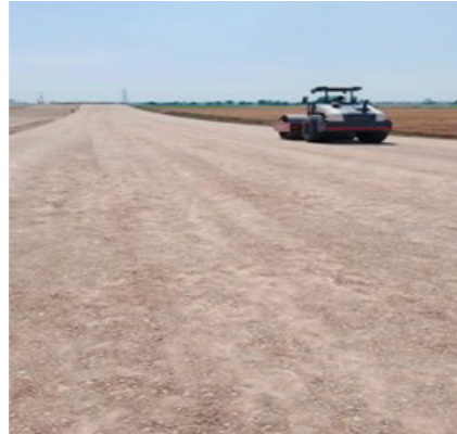
Construction of 4-Lane Greenfield Jalbehra – Shahbad section of NH-152G
