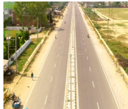
Construction of four-lane Greenfield Amritsar connectivity
