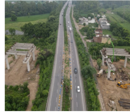
Construction of Four/Six Lane Greenfield Ludhiana-Rupnagar NH-205K
