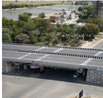
Construction of 6-lane Greenfield Varanasi-Ranchi-Kolkata Highway (Package 11)
