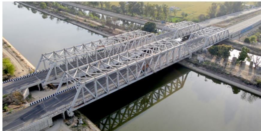
Flyovers and Bridges
