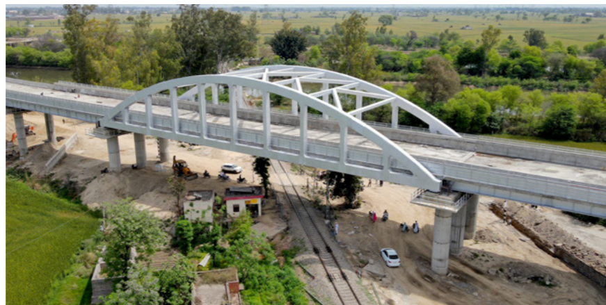
Rail Over Bridges (ROB)
