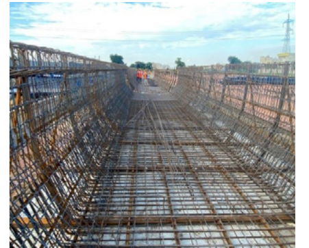
Design and Construction of Agra Metro elevated viaduct and stations
