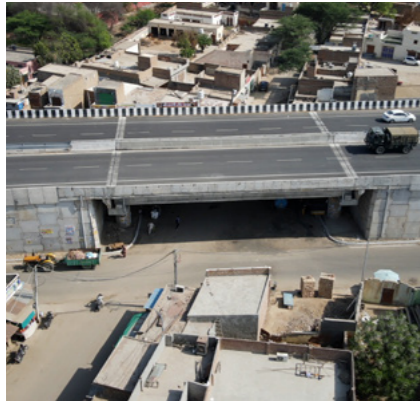
Construction of 6-lane Greenfield Varanasi-Ranchi-Kolkata Highway (Package 12)
